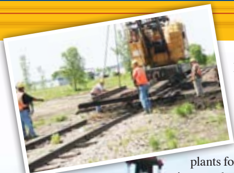
Gang 2915 employees place new panels on the Albert Lea Subdivision's Ventura Industrial Lead.
